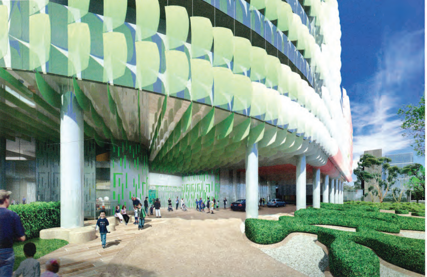
Figure 2. Visitors enter the building via a “treetop canopy” created by more than 1,000 large leaves of shimmering glass, which act as a sunshade for this western façade.
