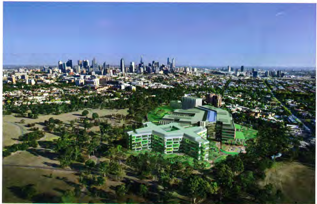
Figure 1. The new Royal Children's Hospital, opening in 2011, in its parkland setting, aims for a 40% reduction in carbon emissions.
